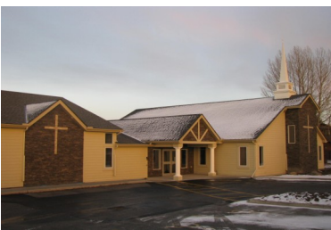
St. Paul Calgary—Renovation Complete!
